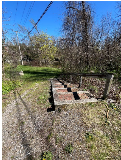
Stairs to Middle Level
