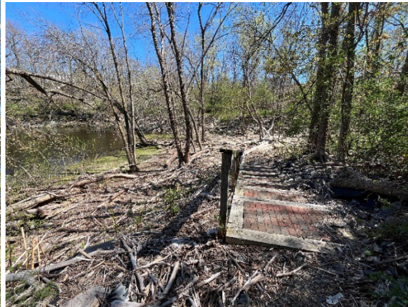
Stairs to Lower Level and River Access
